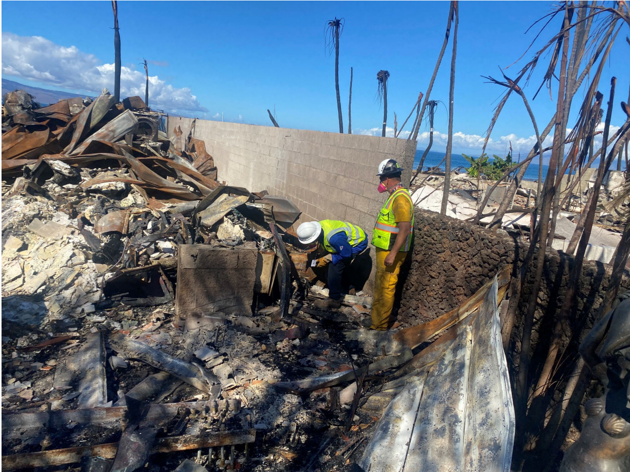
Residential Battery Energy Storage System
